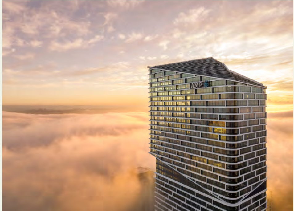
Quay Quarter Tower. Photo credit: Adam Mork
