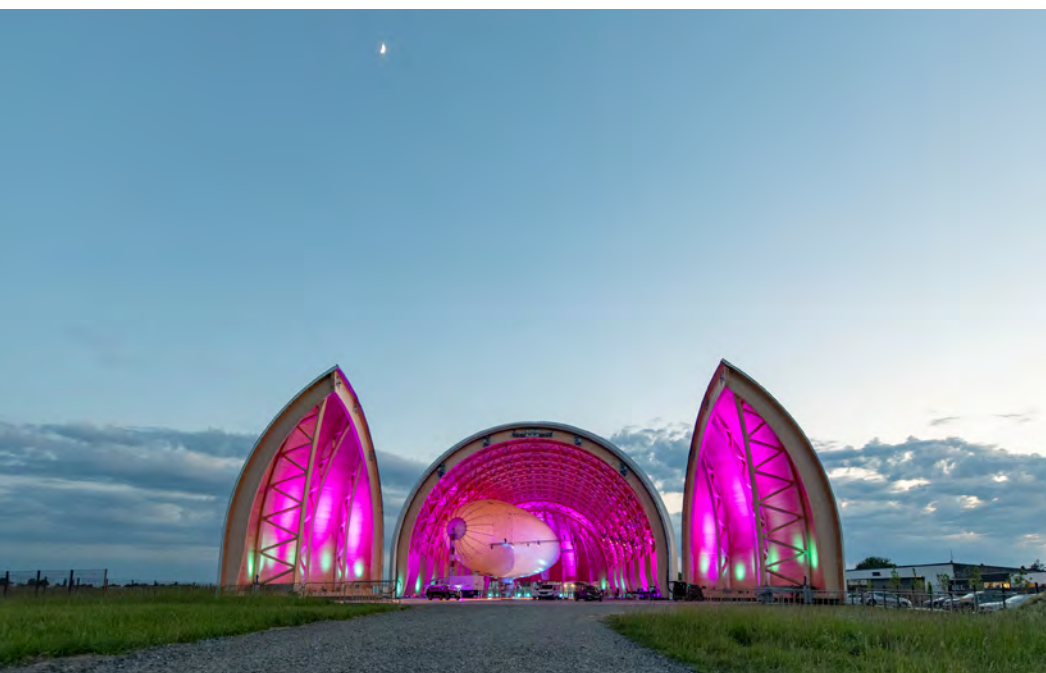
The Mülheim airship hangar in Germany combines innovation, sustainability, and a pioneering spirit to create a breathtaking piece of modern architecture. Copyright: Stefan Lamberty / WDL
