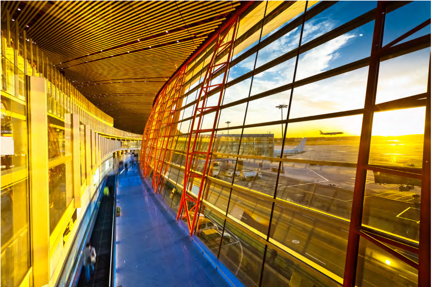
Beijing Capital International Airport Terminals T3A and T3B. The airport construction used over 8,000 tonnes of steel, much of which is coated with Hempel.
