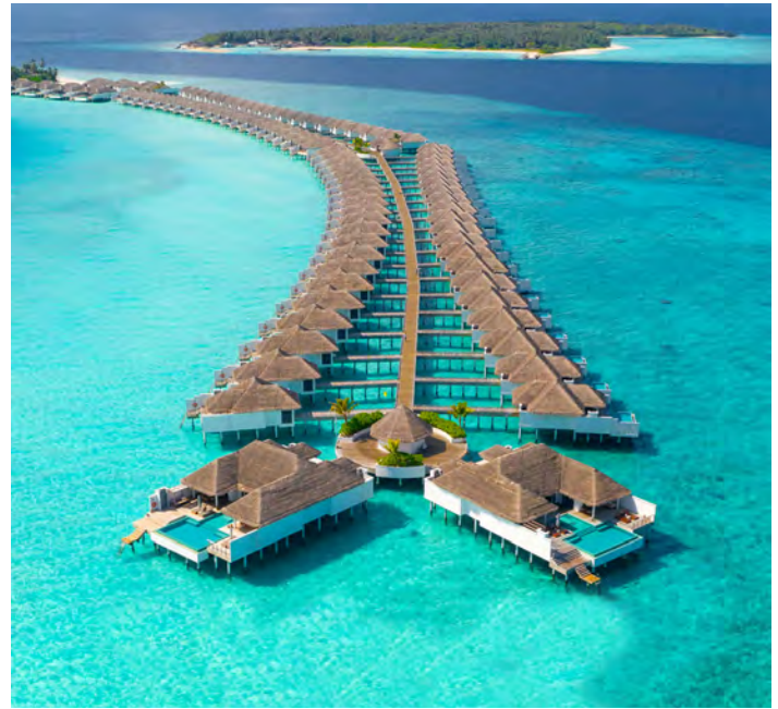
Finolhu Renovation Project
